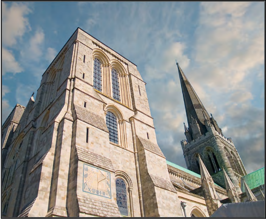
Fig 8.9 the completed image.
